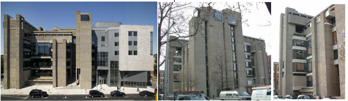
Art and Architecture Building, Yale (1958-1964) (耶魯大學建築系館) / Paul Rudolph
