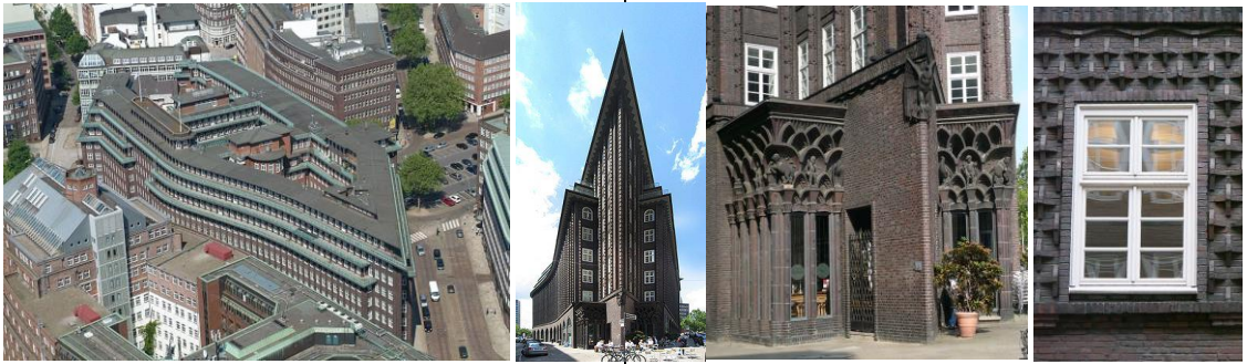
Chilehaus in Hamburg by Fritz Höger (1923)
