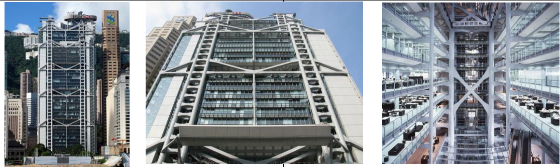
HSBC Building, Hong Kong (香港匯豐銀行大樓) (1985) /Norman Foster
